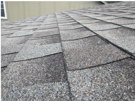
Raised section of sub roof
