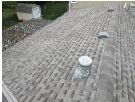
roof covering in good condition
