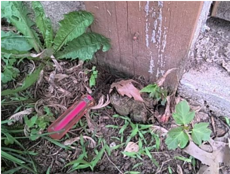
wood rot on posts in contact with soil
