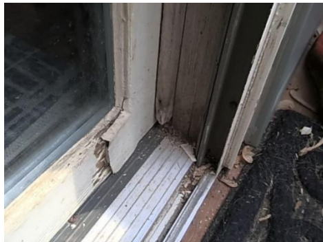
damage to rear slider, exposed wood frame
