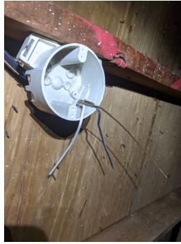
improperly terminated wiring in the attic
