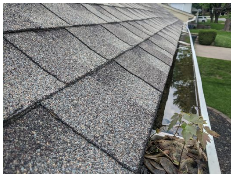
The front gutter was restricted and full of water
